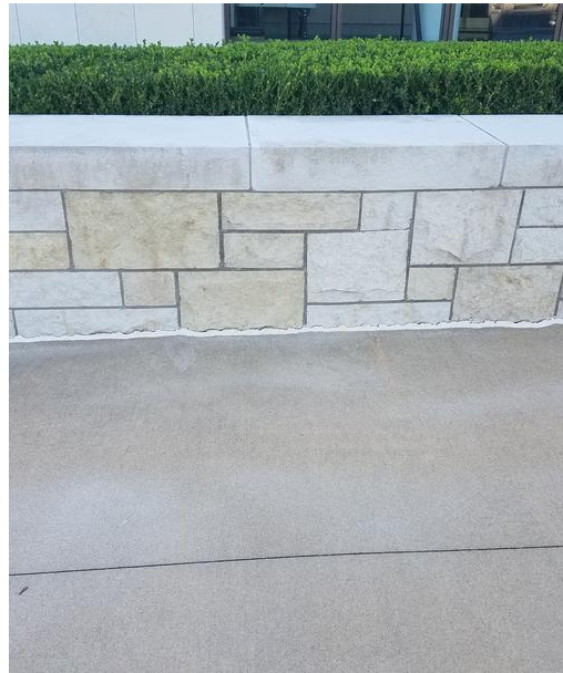
Exterior Walls and Ledges
